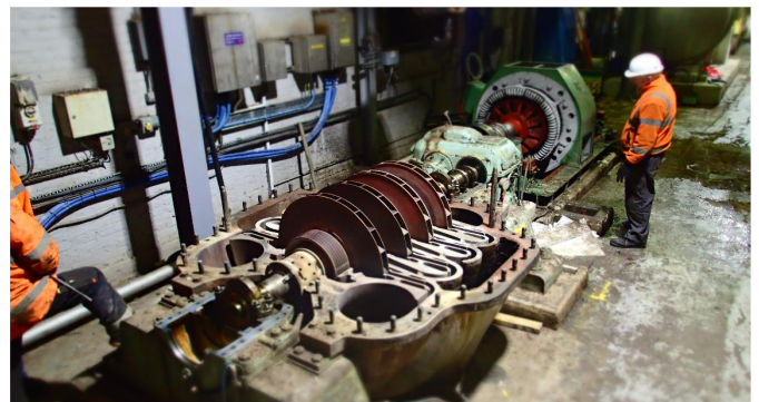
Dismantling old blowers
